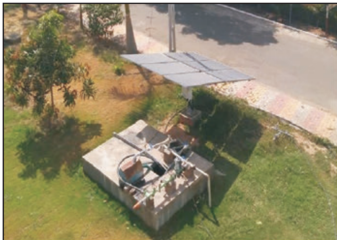
Solar Water Pumping System
