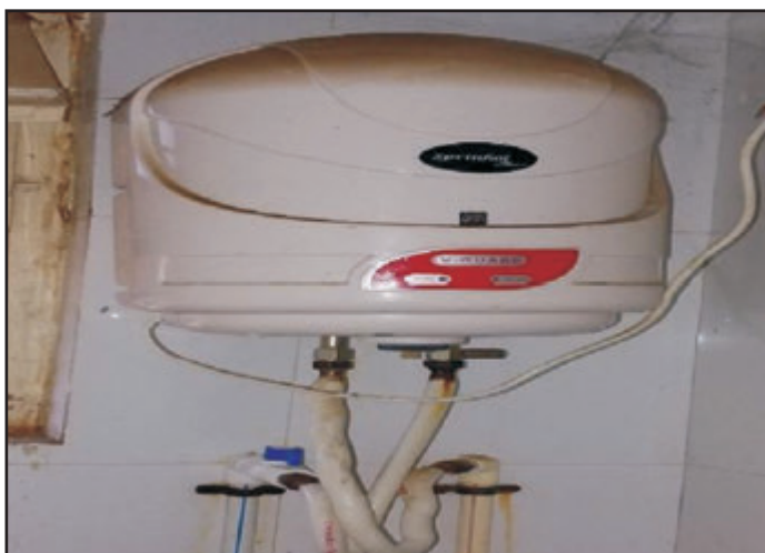
Electric Geyser for water heating
