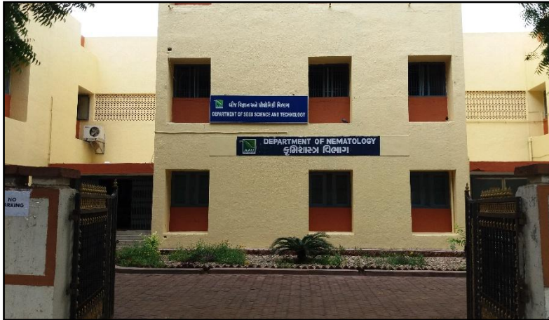
Deptment of Seed Science and Technology Building
