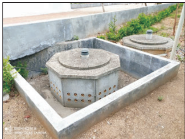
Rooftop Water Harvesting Structure
