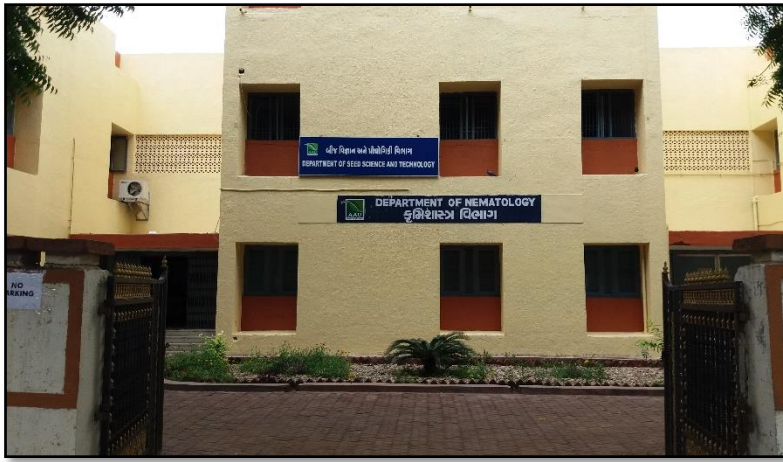
Deptment of Seed Science and Technology Building
