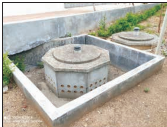
Rooftop Water Harvesting Structure
