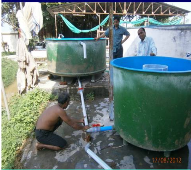
For automatic egg collection Intervention made by AAU, Fisheries Scientists – Reinstallation of FRP carp hatchery
